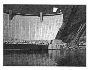
Glen Canyon Dam discharging 8,000 cubic feet per second (cfs), March 25, 1996 (from US Geological Survey's Web Page).
