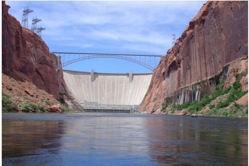
Figure 3. Glen Canyon Dam.
