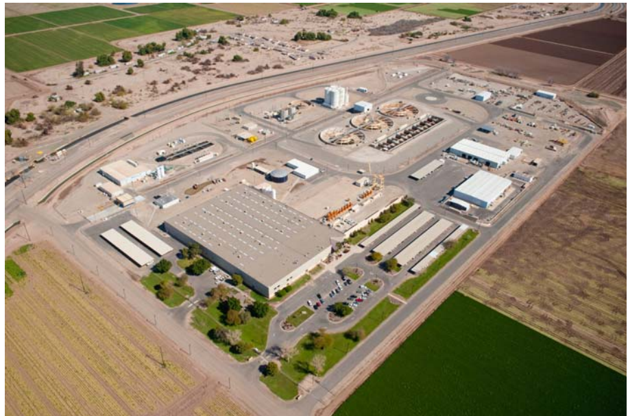
Aerial photo of the Yuma Area Office and the Yuma Desalting Plant. Photo credit: Andrew Pernick; Bureau of Reclamation.
