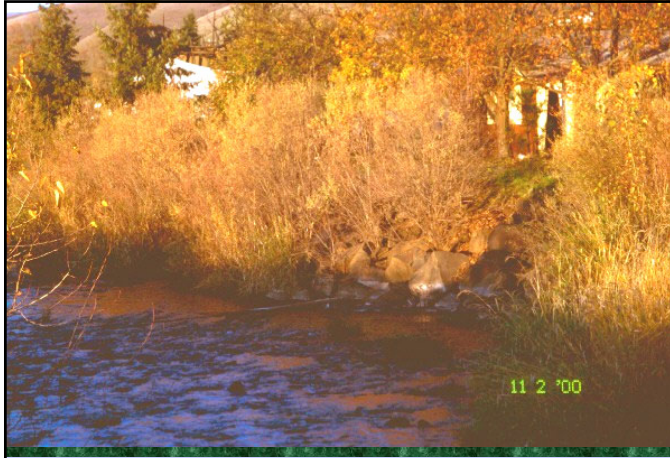
Rock rip-rap area with poles in ecosoil as of 2000, planted in 1998
