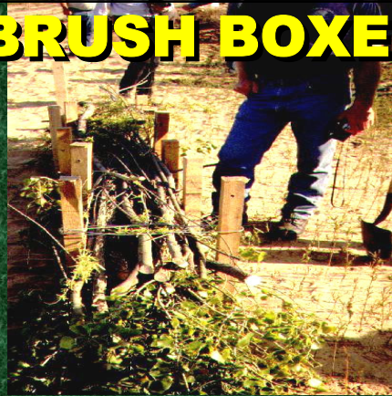
BRUSH BOX BREAKWATER
